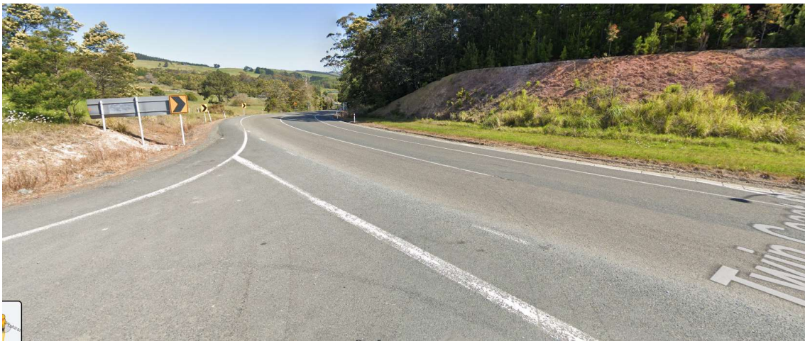
Figure 8: Looking left from Tuhirangi Road onto SH16 – Google Map Street View
