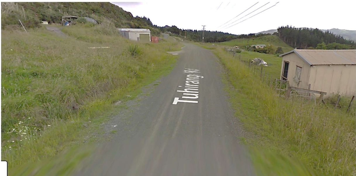
Figure 4: Existing Tuhirangi Road
